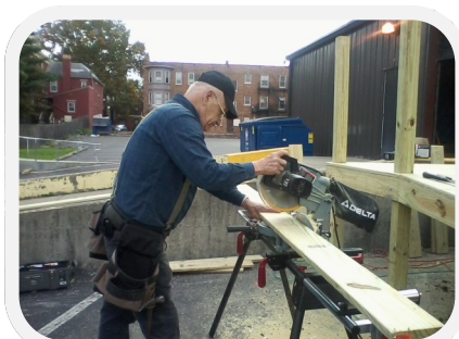
Master Carpenter, Larry Sendelbach cuts with great precision
